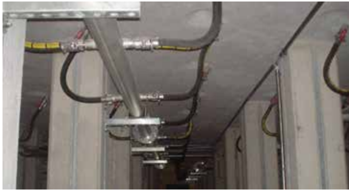
Service room beneath the digester vessel
